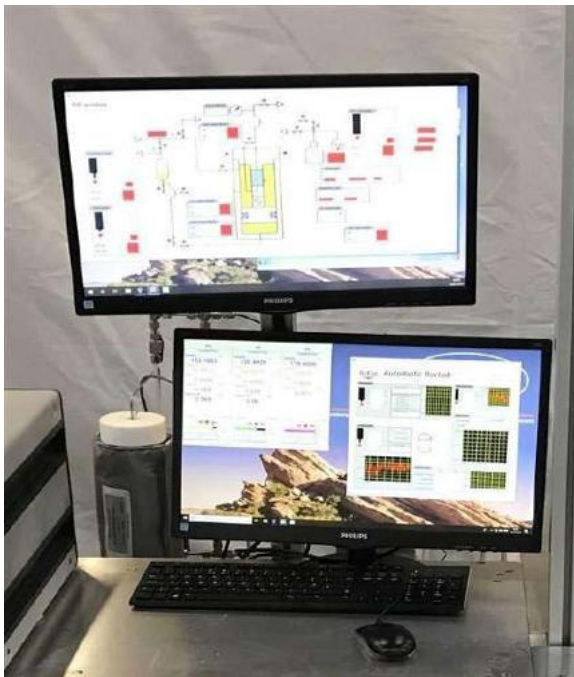
Dual-screen control station — synoptic + acquisition
